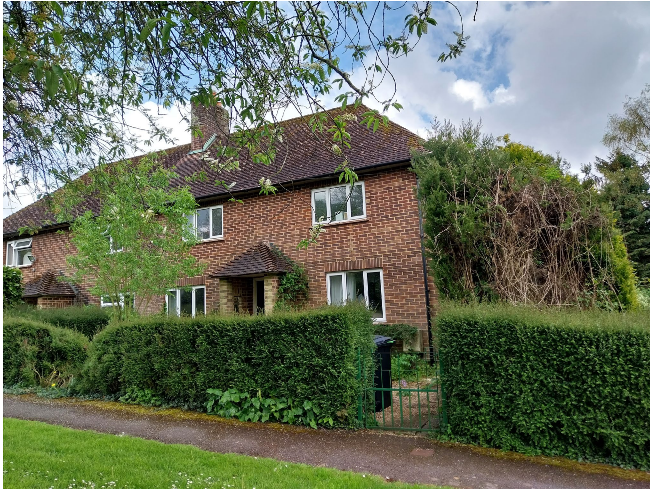
Photo Front elevation of property
